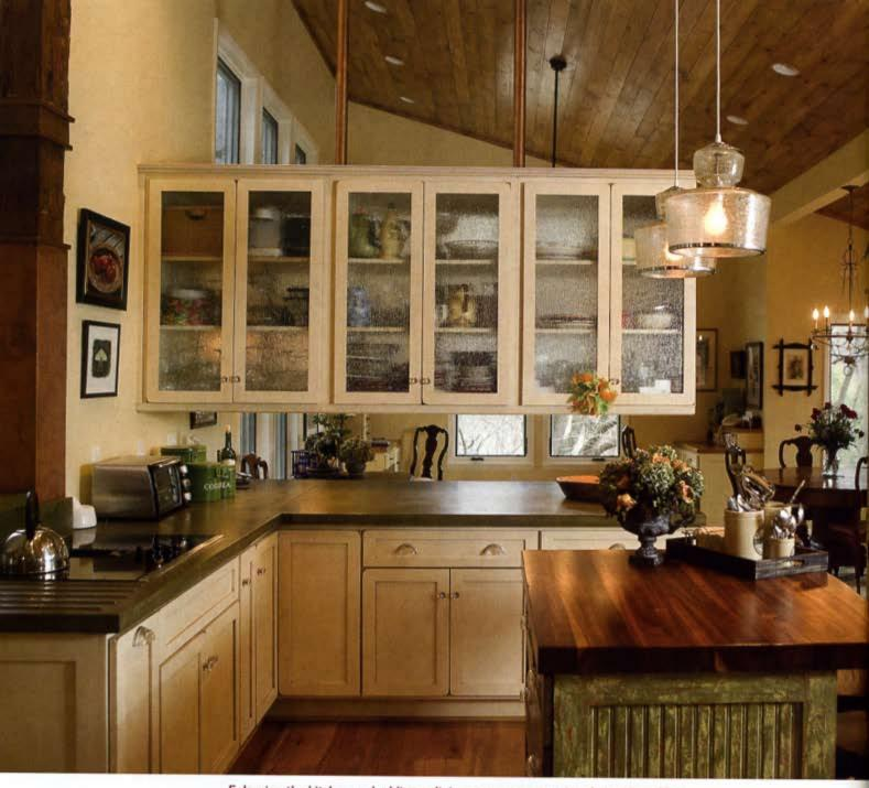
Enlarging the kitchen and adding a dining room meant raising the roofline. The weight of the hanging cupboard between kitchen and dining room is borne by rafters in the ceiling and reinforced with galvanized steel pipes and strategically placed steel plates. The distressed cabinets are by West End Cabinets.
